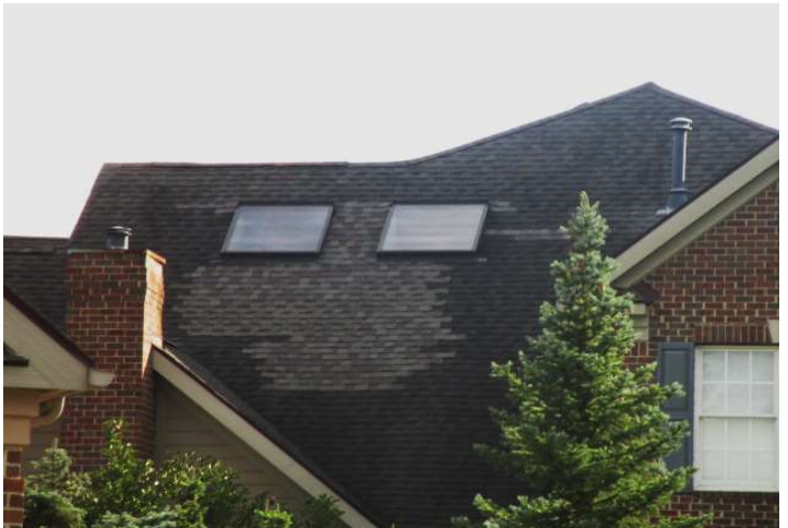
Patch on asphalt shingles roof
