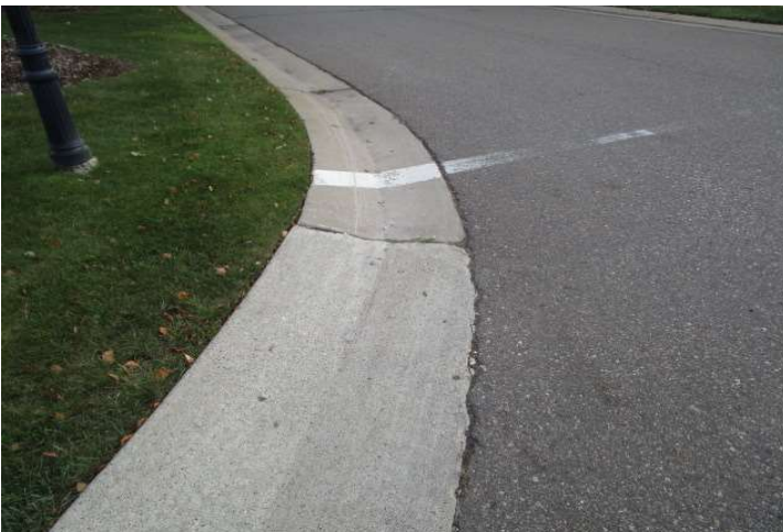
Concrete curb and gutter
