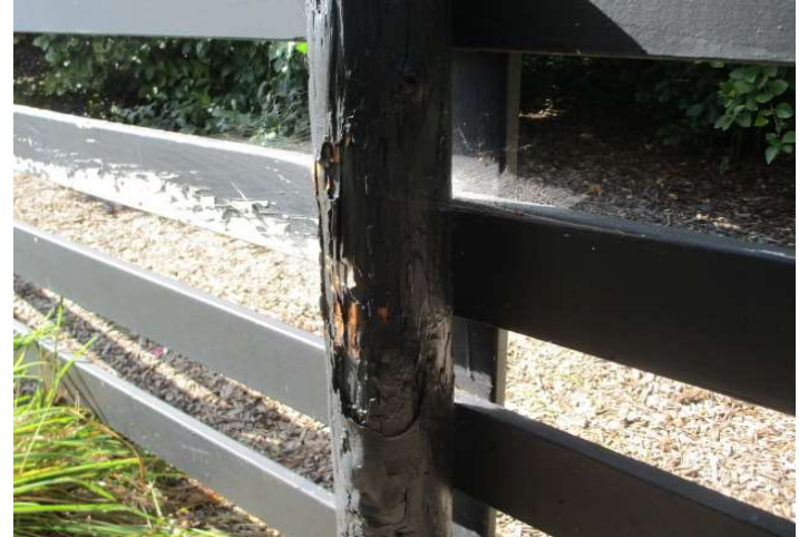
Chips in paint finishes and rotted wood
