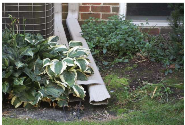
Dented downspout
