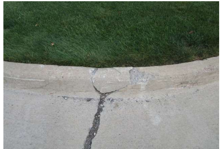
Crack in concrete curb
