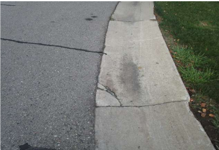
Crack in concrete gutter
