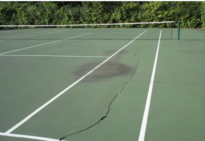
Tennis court with discolored area and crack
