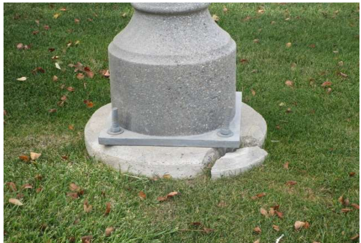
Base of the light pole with chip in concrete
