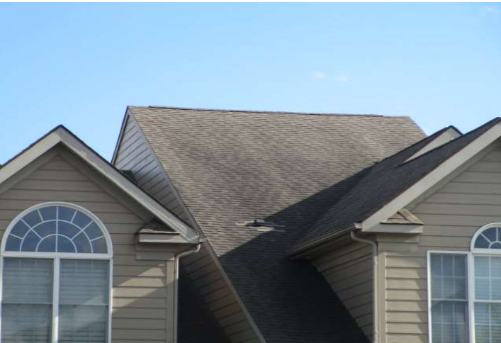
Patch on asphalt shingles roof
