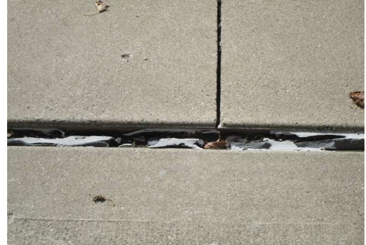
Tripping hazard at pool concrete
