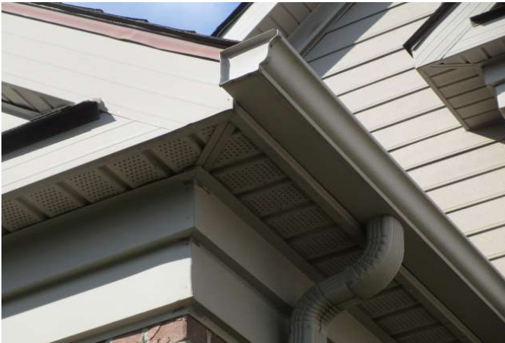
Gutter and downspout connection
