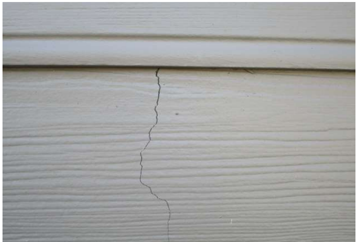
Composite siding with crack
