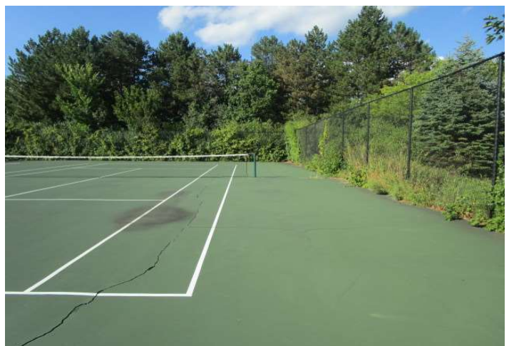
Tennis court with discolored area and crack
