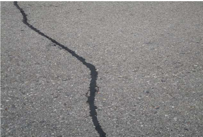
Crack repair on asphalt pavement
