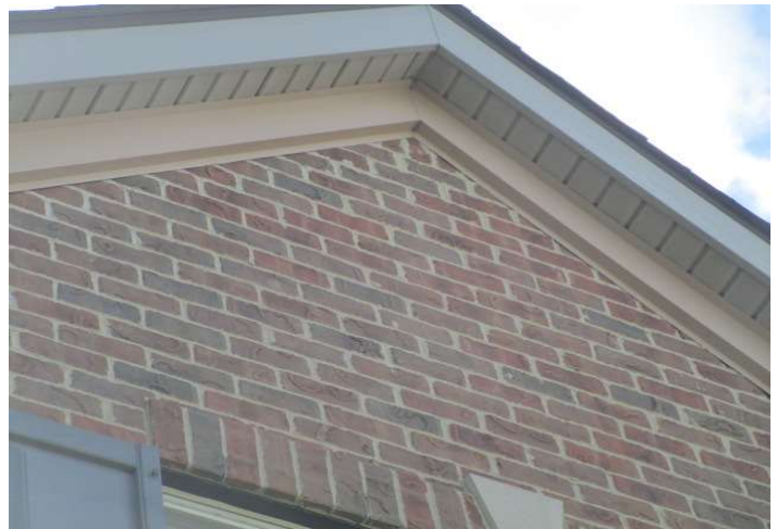
Soffits and fascia at roof
