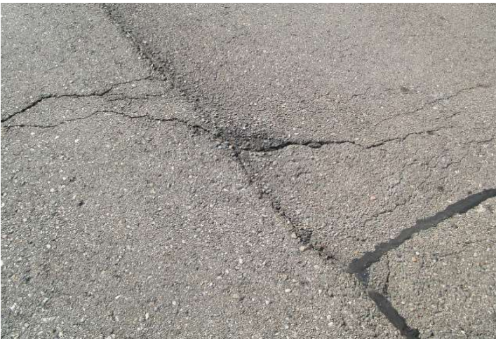
Asphalt pavement street with cracks
