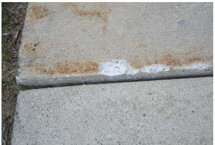
Chip in concrete sidewalk
