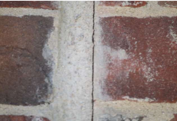
Crack in mortar
