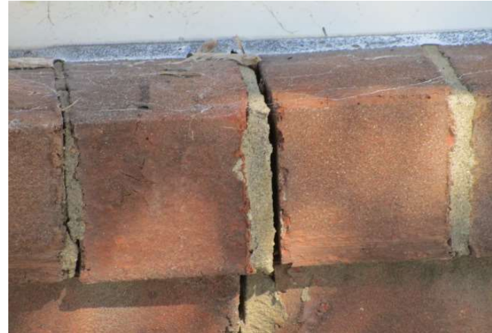
Crack in mortar
