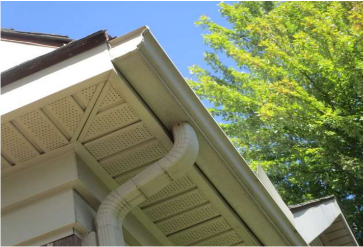
Gutter and Downspout connection
