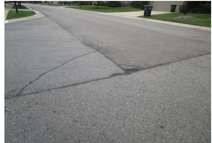
Asphalt pavement street with cracks
