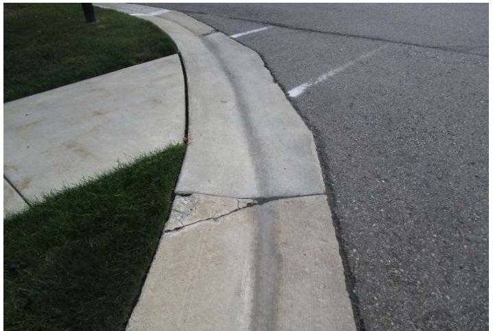
Crack in concrete curb
