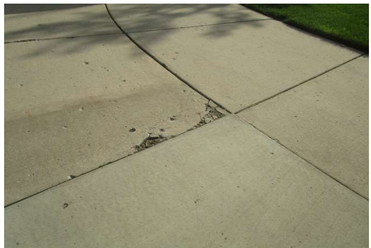
Cracks in concrete driveway
