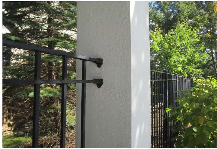
Steel pool fence attached to gazebo
