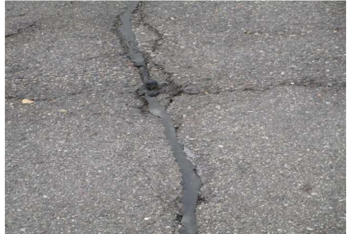
Crack in asphalt pavement
